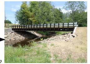
The finished, 65 foot long, spread footer bridge at Daniels Road in South Canaan Township
